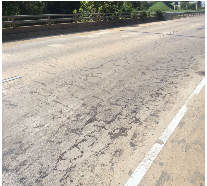
PHOTO 2 Description The driving surface of the deck has sealable cracking.
