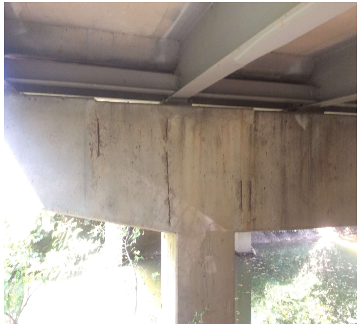
PHOTO 2 Description Span 3 side of Bent 3 cap has delaminated areas and shallow spalling with exposed reinforcing steel where steel was placed against the forms during the construction process.
