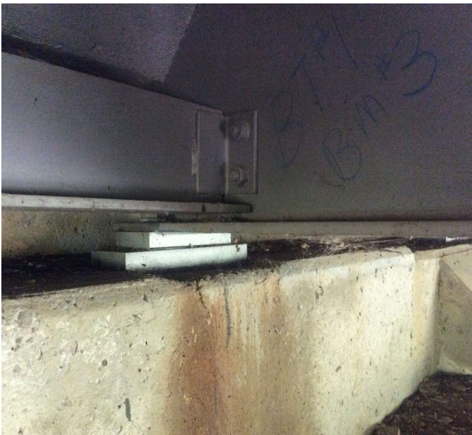
PHOTO 1 Description Bearings have fine metal powder between the masonry plates and the sole plates indicating excessive movement during traffic impacts. Visible (Approximately 1/16") movement in the bearing at Bent 1, Beam 3 during traffic impact at this inspection.
