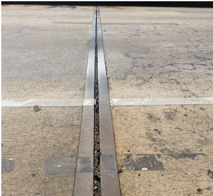
PHOTO 1 Description Compression seals are deteriorated and torn in locations.
