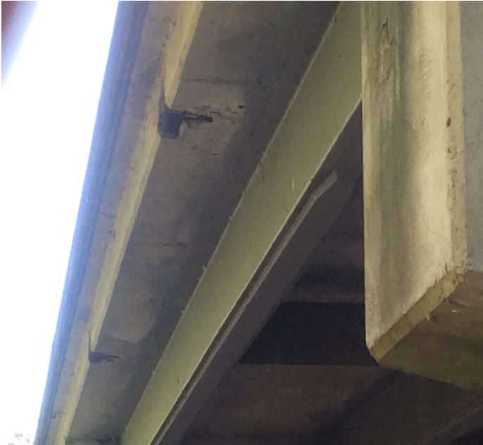
PHOTO 3 Description The overhang portion of the deck on the Lt side has spalling with exposed reinforcing steel adjacent to deck drains.
