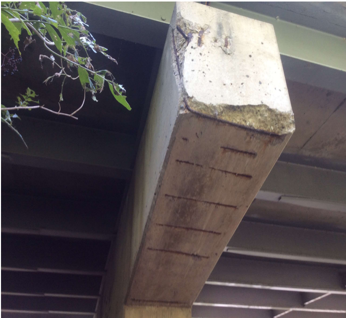
PHOTO 4 Description The undersurface of Bent 3 cap has shallow spalls with exposed reinforcing steel outside both columns. Exposed reinforcing steel appears to be #4 bands that have up to initial section loss.
