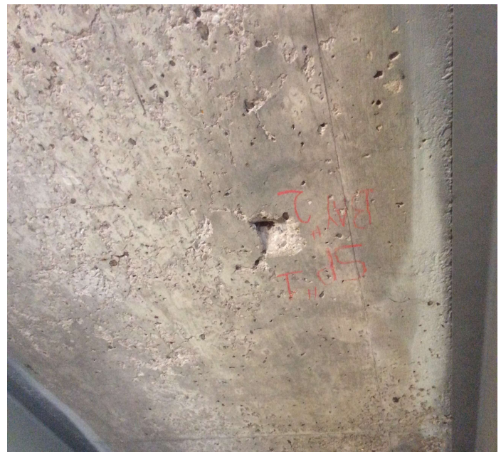
PHOTO 2 Description The undersurface of the deck in Bay 2 of Span 1 has an area of spalling with exposed reinforcing steel.
