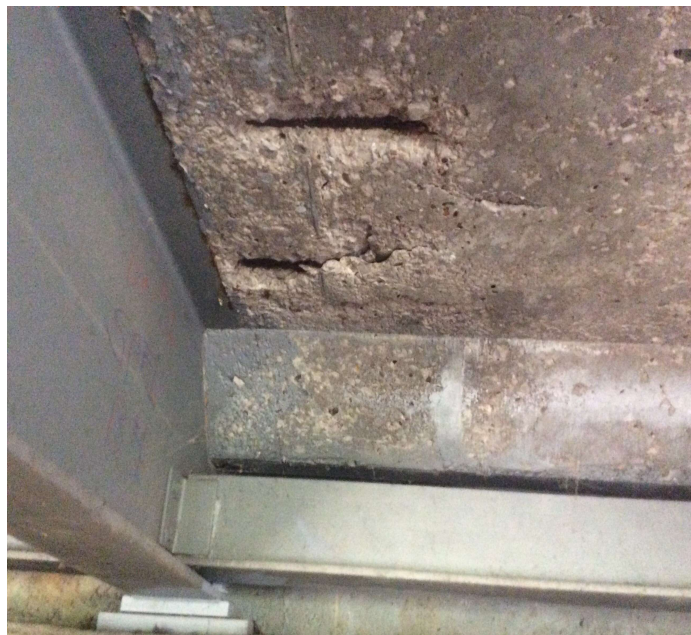
PHOTO 1 Description The undersurface of the deck in Bay 1 of Span 1 near the South abutment has an area of spalling with exposed reinforcing steel with the area surrounding the spall is delaminated in locations.
