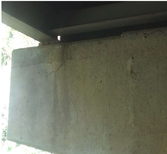
PHOTO 1 Description The Lt end of Bent 2 cap has a 4' long horizontal crack located approximately 8" below the top of cap.
