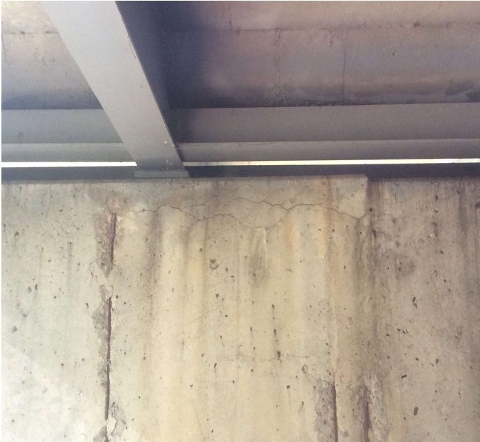
PHOTO 3 Description There is a 3' area of map cracking in the bearing area of Beam 6.
