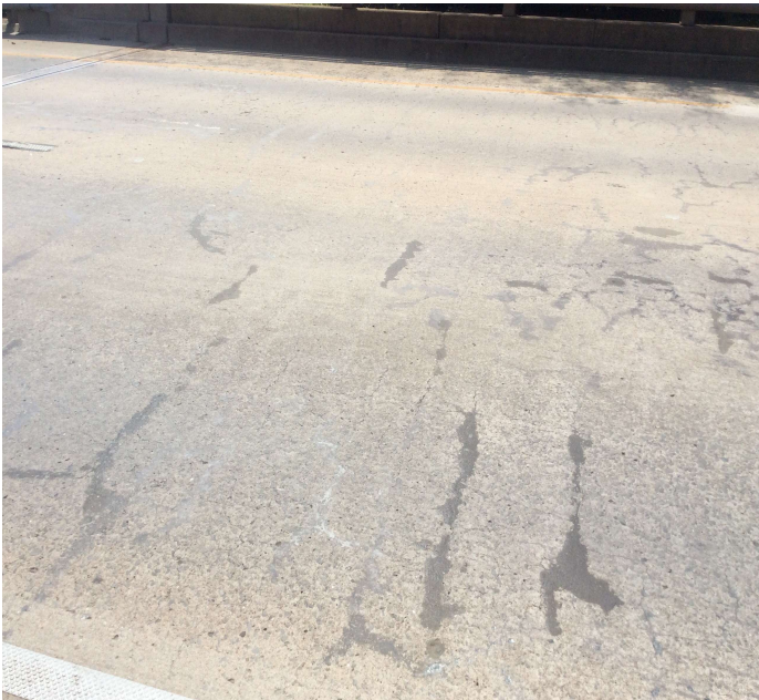
PHOTO 1 Description The driving surface of the deck has sealable cracking.
