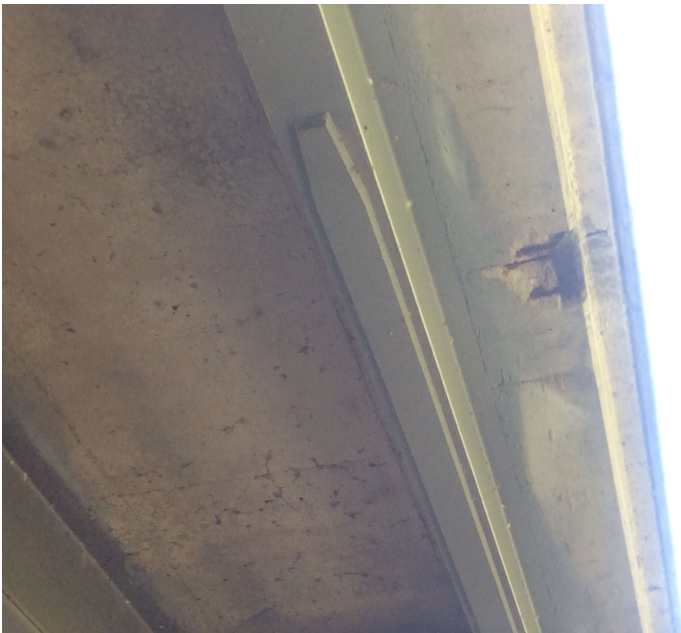
PHOTO 4 Description The overhang portion of the deck on the Lt side has spalling with exposed reinforcing steel adjacent to deck drains.
